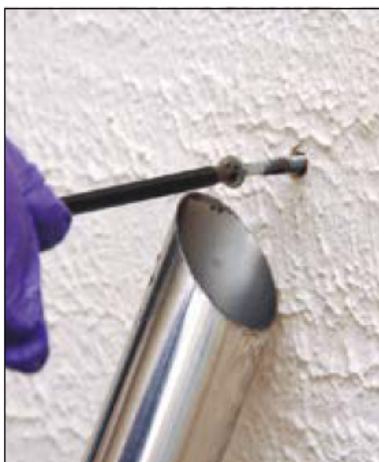
Control measures: shadow vacuuming and using a drill cowl as local extraction (圖片來源：英國HSE)
