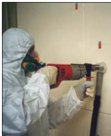
Control measures: shadow vacuuming and using a drill cowl as local extraction (圖片來源：英國HSE)
